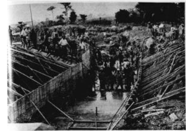
The Incheon Key Drain at Kumasi in process of construction.
